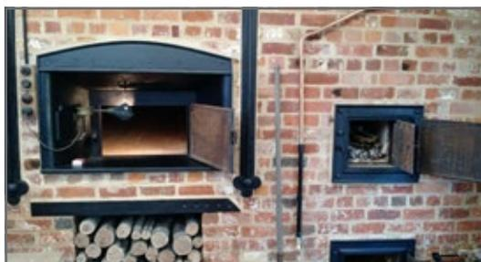
The pre-firing photo shows the oven to the left with new fire bricks installed on the floor. It is lit by a lamp which is the original left in place. To the right is the fire set and ready to go.
